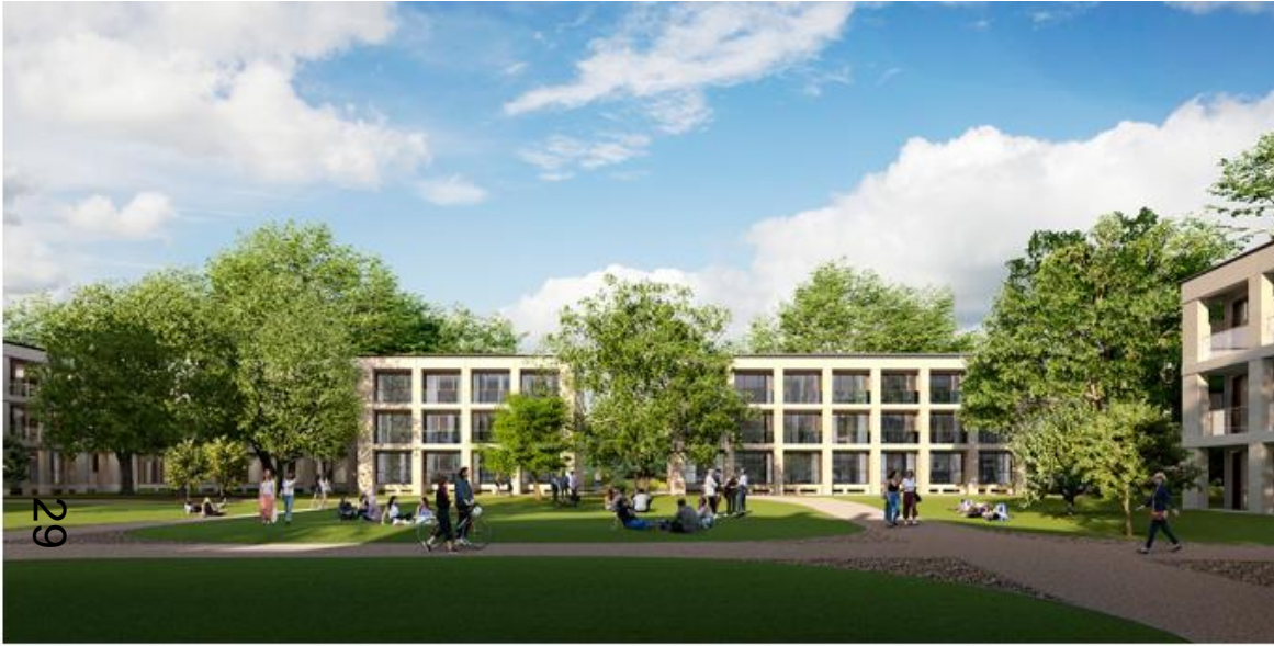
Indicative view looking across the Great Court towards the new Great Court West student accommodation building
